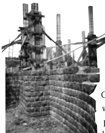
Current construction work on the Archives, Museum, and Research Building.
