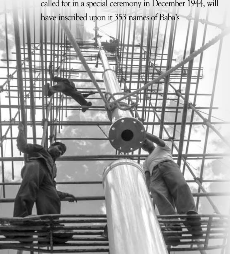
Recent installation of the central steel pipe.
